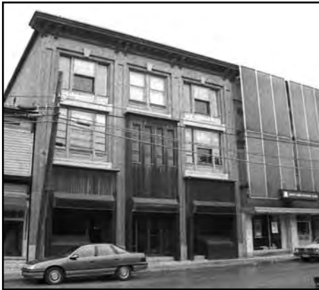
The Greenberg Building and Union National Bank in 1987. Our building had a California redwood façade, and the bank had an “aluminum cheese grater” façade.
