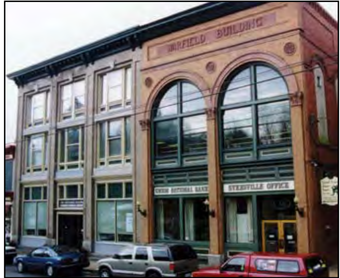
The Greenberg Building and Union National Bank in 1995 with restoration of their traditional facades.
