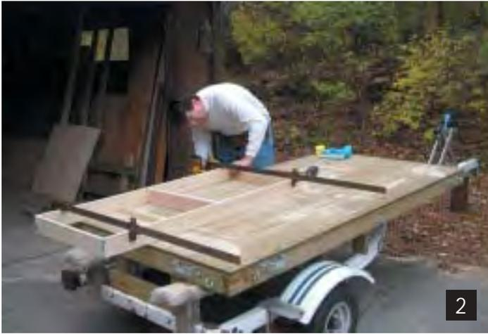
**Photo 2** shows the basic set up for creating the frames. I pre-drilled and then screwed the pieces of the frame together using large bar clamps for accurate positioning. This task is much easier to do with a cordless drill that has interchangeable bits for drilling pilot holes and driving screws.
