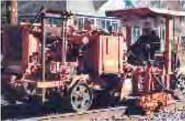
6. An Anchor-Spreader followed next, removing the loose metal plates located between the rails and ties.
