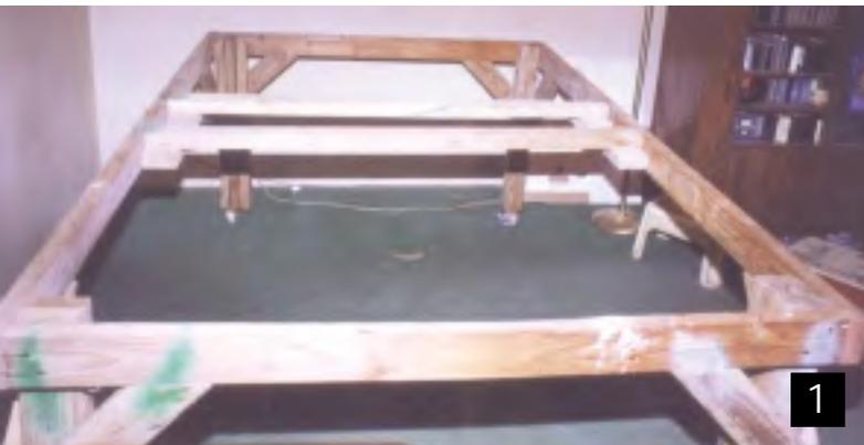
work as seen in **photo 1**. Casters were installed on the bottom of the four legs so that the bench frame could be moved around, allowing access to all areas of the train garden.
