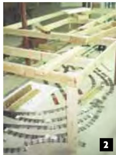
The benchwork is constructed over track temporarily “installed” on the floor.
