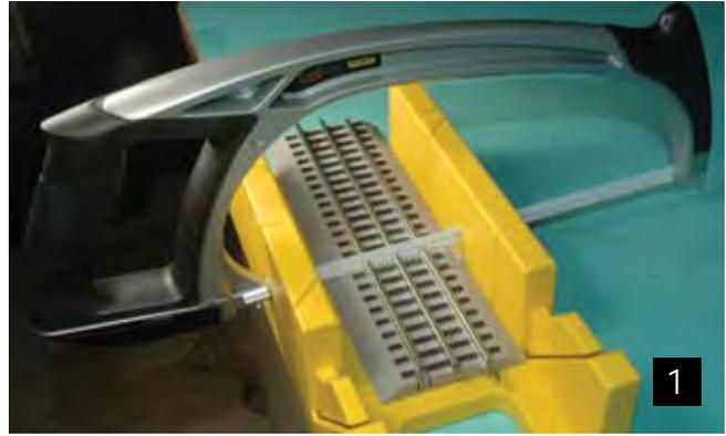
**Photo 1** shows the setup as the sawing proceeds. You must hold the track firmly while sawing. Once you get through the metal rails, the cutting will go quickly. After the first cut was made, I positioned the two pieces as shown in
