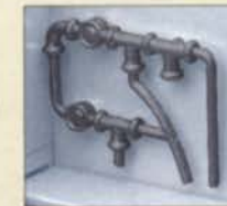
Separately applied piping
