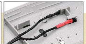
Wire attached to terminal
