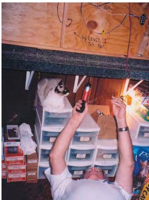
All wiring is installed underneath the platforms in harnesses and brought up from underneath to each lock-on or accessory. Four Lionel KWs provide track and accessory power to the platforms, and smaller transformers provide power for lighting. Maximillian “assists” Mike in stringing a bus wire for lighting the structures along the south wall.
