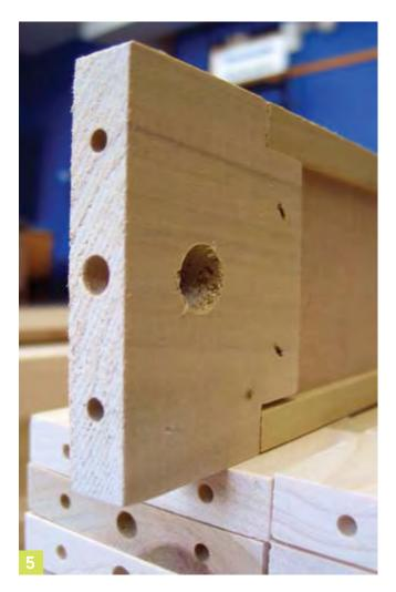
The beams which make the actual benchwork are unique in their design. Rather than solid wood, each beam is constructed with five pieces of wood. **Photo 5** shows the end of one of the beams. The center section of the beam is ½-inch medium density fiberboard (MDF). This piece is capped on its two long edges with poplar strips grooved to accept
