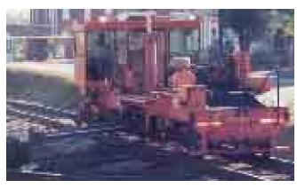
10. A Tie-Remover-Inserter (TRI) now inserts the new ties under the metal track rails. Another TRI adjusted the ties and aligned them correctly under the rails.
