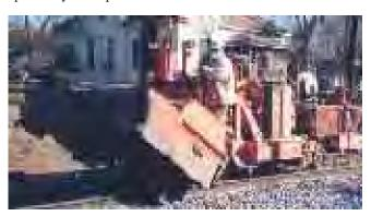
2. A Track Broom Car (TBC) was next in line. The TBC sweeper removed the rocks and dirt from the ties that were to be replaced. Not all the ties were being replaced.
