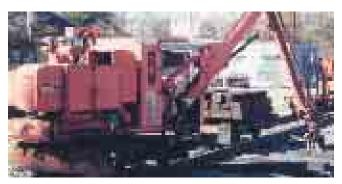
9. New ties are placed in position perpendicular to the rails, ready for insertion.
