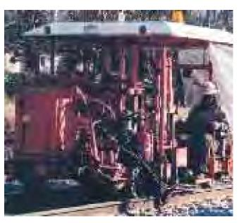
4. Another Spike Puller pulled the spikes located on the outside of the rails, out of the anchors and ties
